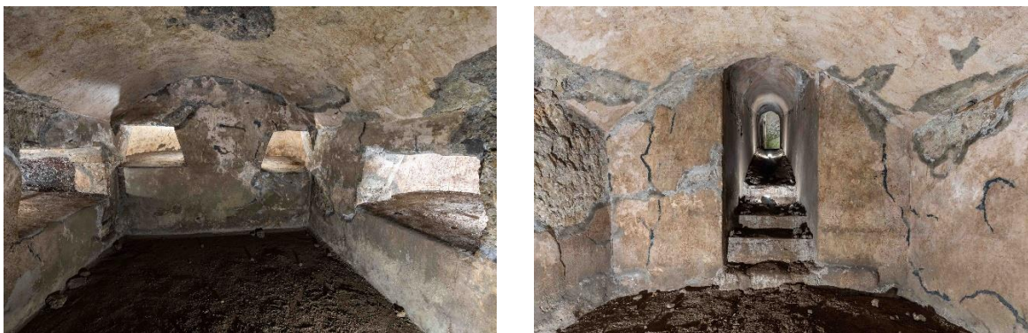
Fig. 15: Cellar under the northern part of the house (left) with access corridor (right); ©Mauro Palumbo
