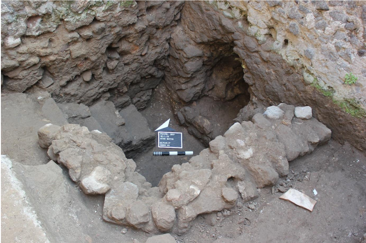
Fig. 3: Area IV, re-excavated subdivision of room with stairs and praefurnium arch towards men's caldarium in the S.
